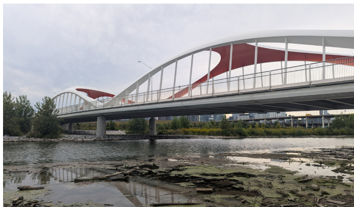
Commissioners Street Bridge passes over new mouth of the river
