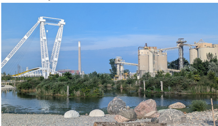
Refurbished Atlas Crane, Amrize silos, canoe launch point
